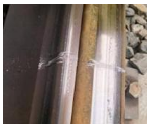
The closed switch rail and stock rail, for measuring the flange drop
